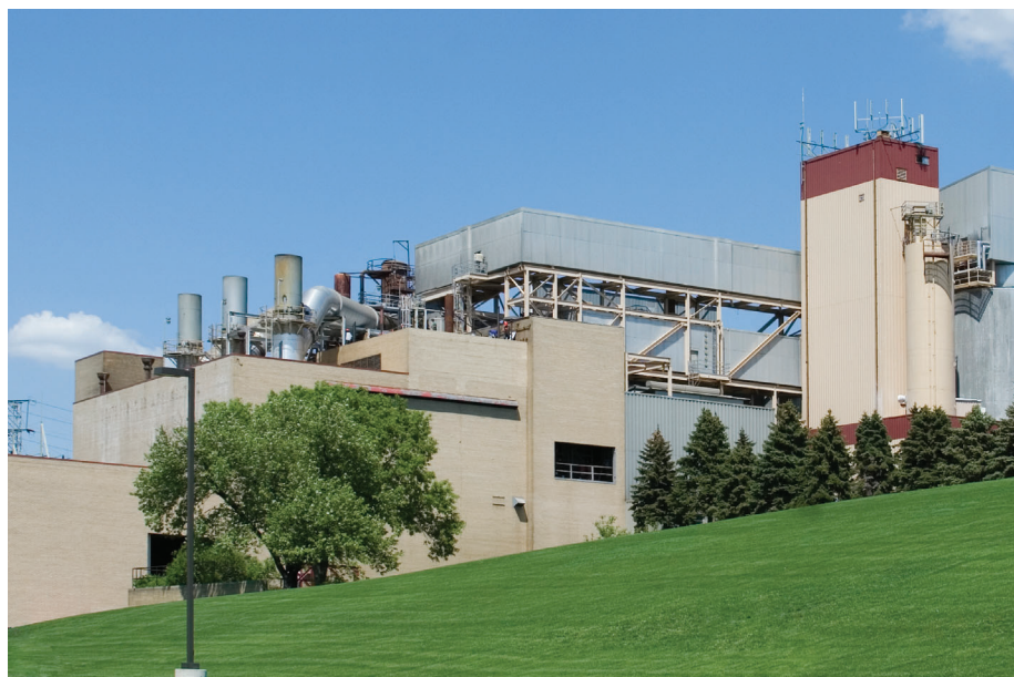
Staff from Great River Energy's Elk River Energy Recovery Station engineered and manufactured a regenerating filter to keep the plant operating without interruption.
