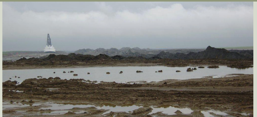
Heavy precipitation and deeper coal seams are leading to additional work and costs Falkirk Mine, the fuel source for Great River Energy's largest power plant.
