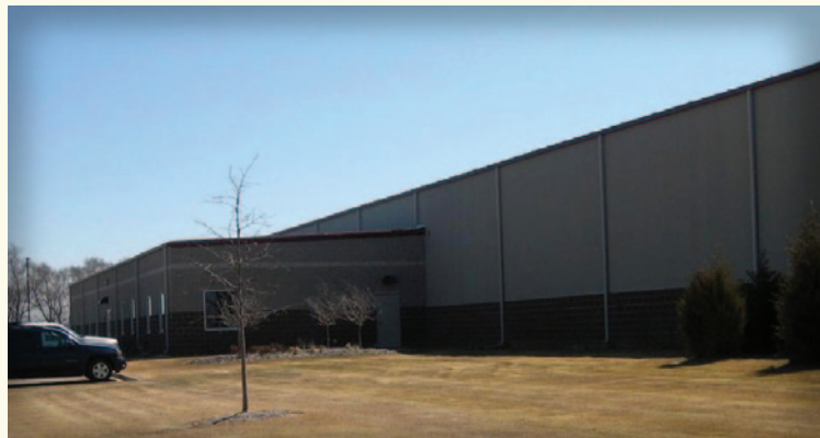
Great River Energy's Big Lake service center is a 41,500-square-foot facility, which opened in May 2008. The building features several energy efficient features, including geothermal heating and cooling. In addition, 34 percent of building materials came from recycled sources, and 24 percent were manufactured locally.
