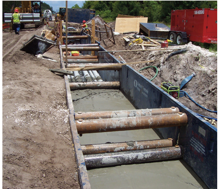
Burying high voltage transmission lines is extremely disruptive to property. An open trench is required throughout the construction process.
