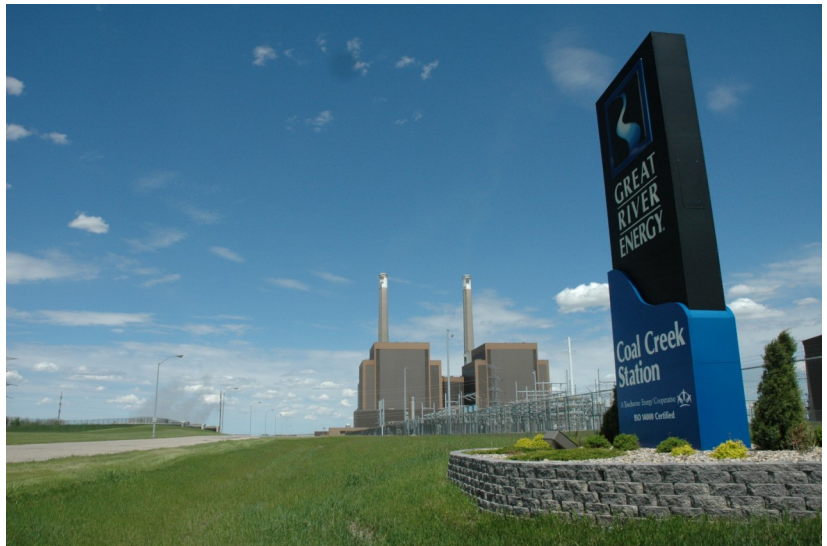
Coal Creek Station near Underwood, ND.
