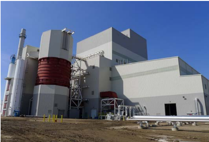
Spiritwood Station will use Best Available Control Technologies to control emissions.
